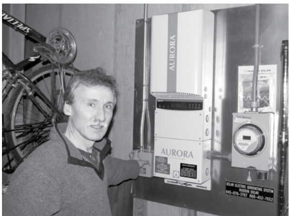
Peter Henderson points to the inverter, which converts direct current generated by rooftop solar panels into alternating current to be used in his home.
