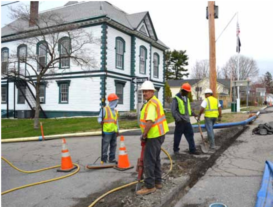
MSI workers Jason Chambers, left, Sergio Leon, Dave Fulford, and Orlando Mejia install a temporary water line near the Philipstown Town Hall, April 10. Photo by J. Tao
