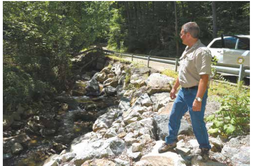
Erosion protection must be rebuilt along this stream on the shoulder of South Mountain Pass Rd.
