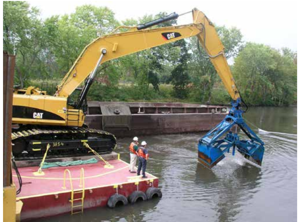
Dredging the Hudson River to remove PCBs
