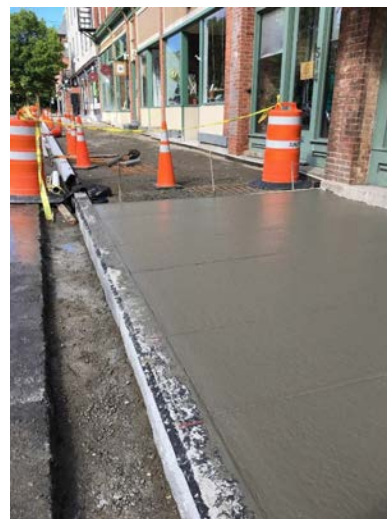
New sidewalks being installed along the east end of Main Street in June 2019.
