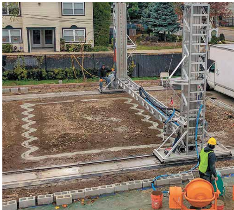
SQ4D tested its 3D house printer on Long Island.
