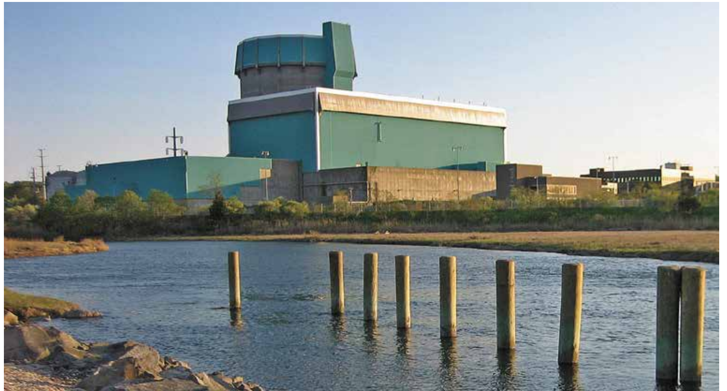
The Shoreham nuclear plant on Long Island was decommissioned in 1994.
