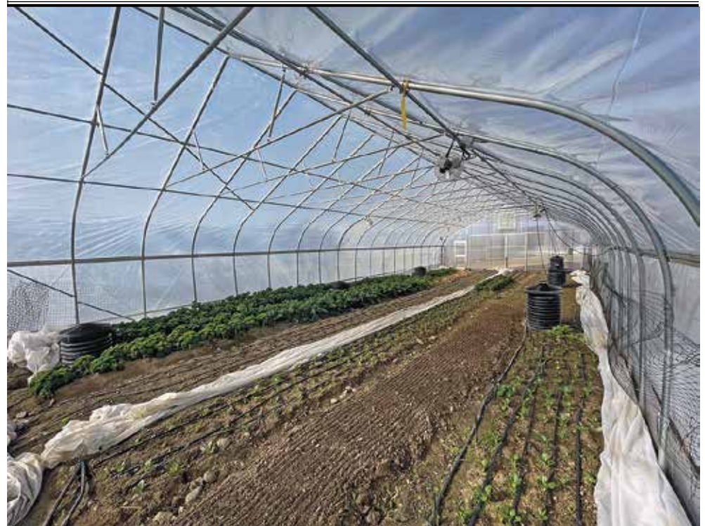
Underground tubes help regulate temperature in this greenhouse at Glynwood. Photo provided
