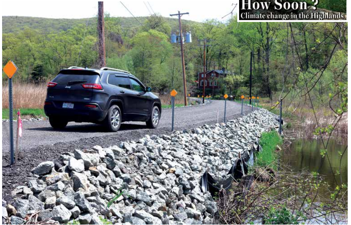
Manitou Station Road in Garrison has been raised 4.5 feet to prevent damage from flooding.
