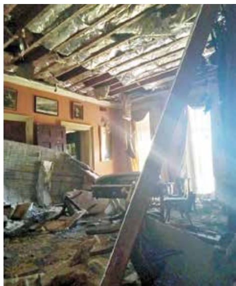
A plaster ceiling collapsed at Boscobel.
