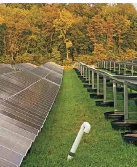
A pipe vents methane from the former landfill at the Beacon Transfer Station, now covered by a solar array. Photo by B. Cronin
