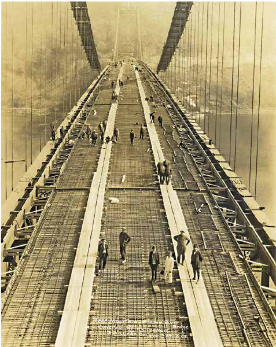
Concrete reinforcement, Oct. 24, 1924
