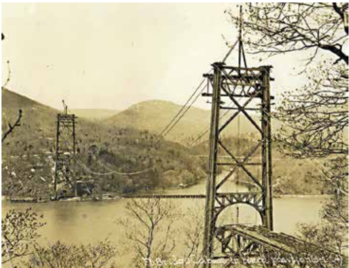
The cables are placed into their final position, May 2, 1924
